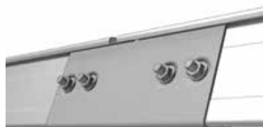
Fasten the connector to the purlins, using four M12x30 bolts, DIN 9021 washers and four M12 flange nuts
